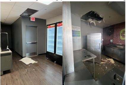
Rainstorm on 10/12 provided a lot of damage inside the building which led to a leak tracking document that is being used to repair continual leaks that have not be resolved. The areas included in these damages were offices, locker rooms, meeting rooms, rubber hallway, and premium areas. Please see photos below which include areas that have already been captured in this document.
